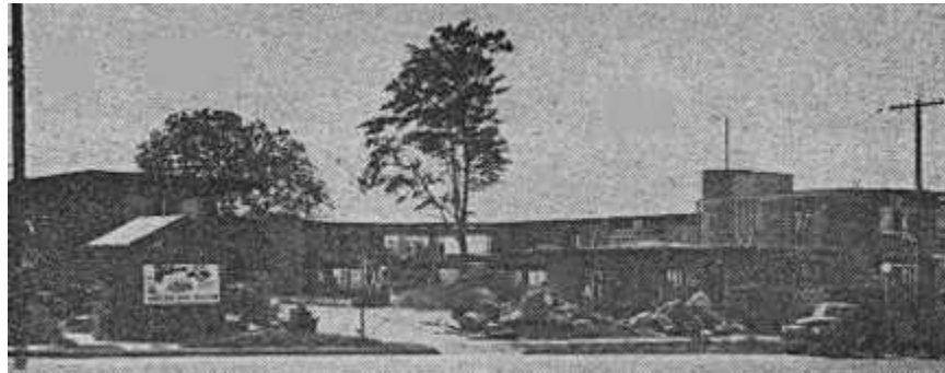
View from US 31 shows front of new, modernistic motel going up at Charlevoix.
